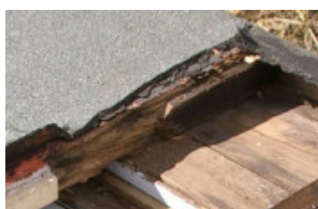
Rotten roof beam
